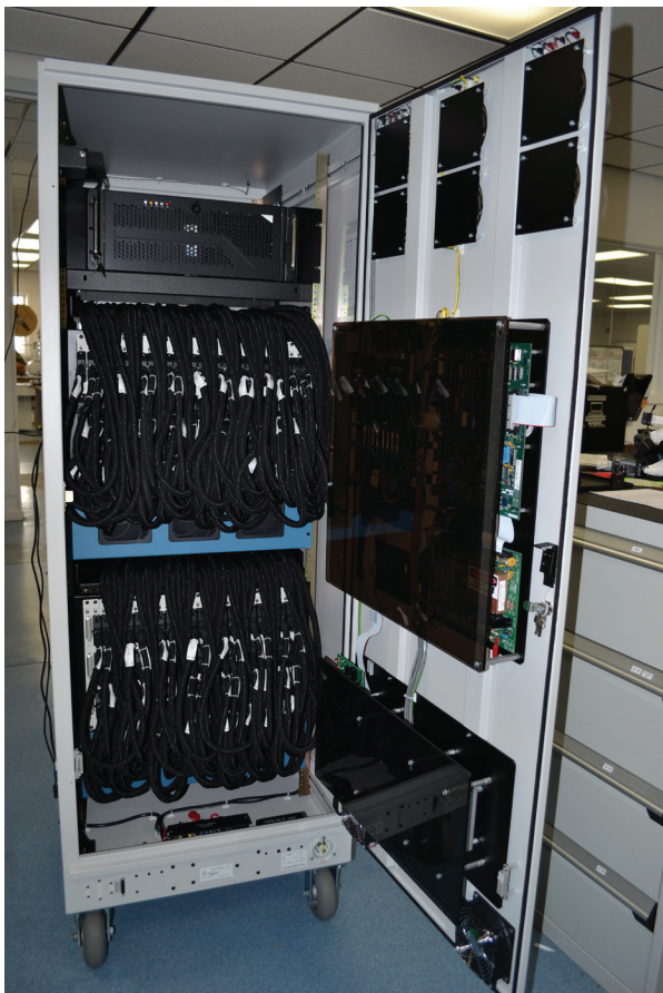
Internal cabling built by VPC's wiring team.
