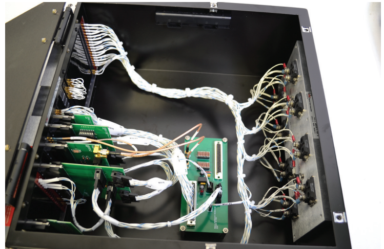
ITA Enclosure with Small PCB Wired to Another PCB
